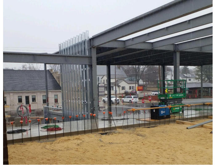
Structural steel going up for addition, main level slab
