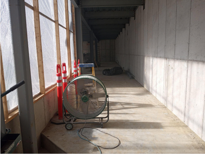
Lower level: looking W into addition from SW corner
